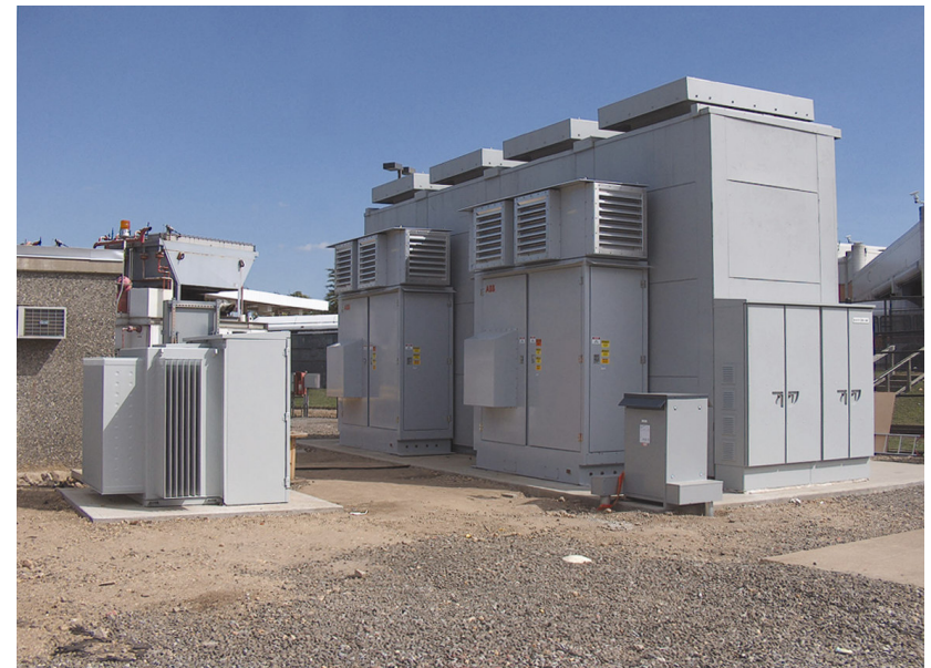
Power Conditioning System Package for BESS
